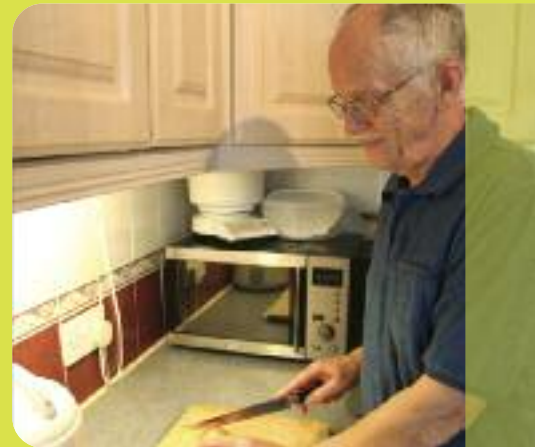
Use of under-cupboard lighting to facilitate kitchen tasks
