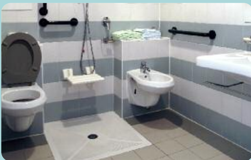
Colour contrast in bathroom to indicate critical surfaces
