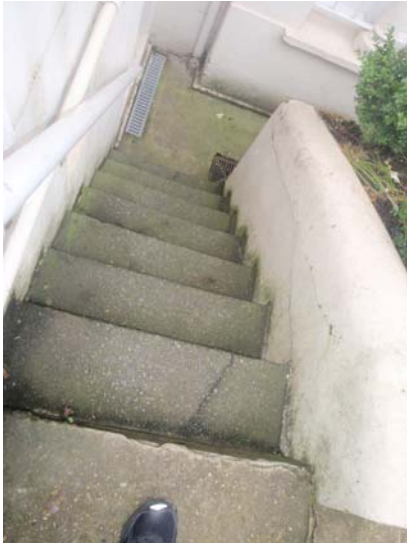
Fig 26 Building 'A' steps and entrance before refurbishment
