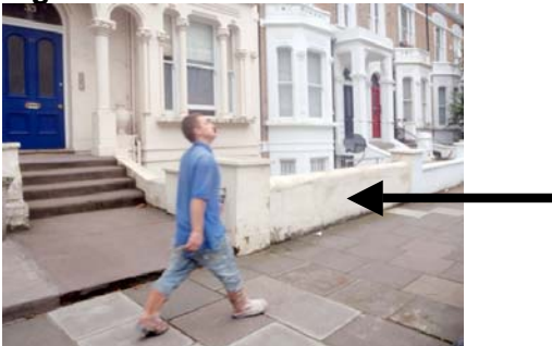
4: Upgrade front wall colour to NCS S1505 Y30R to brighten the façade for visibility
