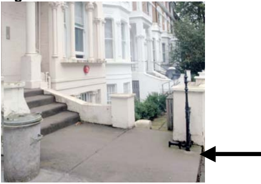
3: Paint step riser/lip black to define change of level with public pavement
