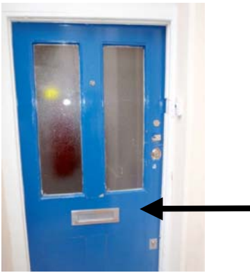
13: Paint front door with NCS S2570 Y90R to contrast with chrome door furniture. (Chrome would provide the highest contrast with a dark door) or replace with a new solid door.
