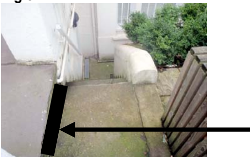
5: Render and paint lip of step dark grey/black to mark the potentially dangerous change of level
